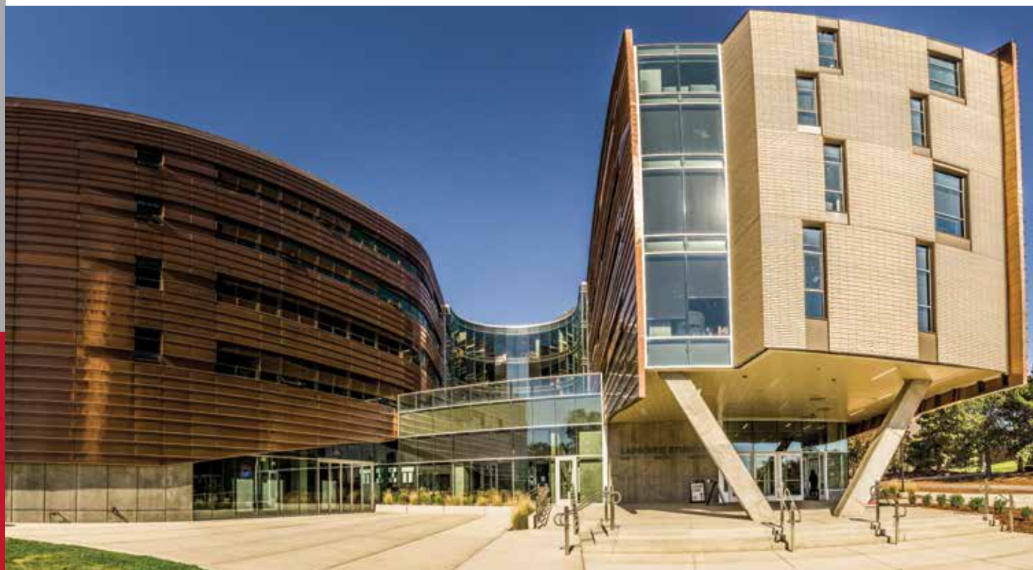
The new copper cladding on the exterior of the Lassonde Studios will change color to a green patina as it weathers over time, mirroring the vibrant, evolving activities taking place inside.
